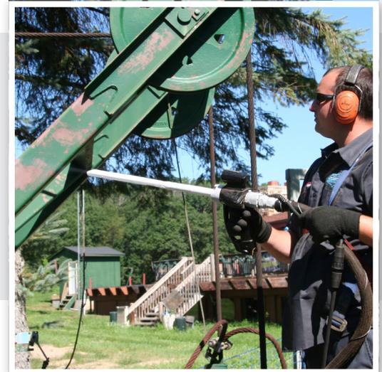
*"OUR EXPERIENCE WITH DRY ICE BLASTING IS THAT IT DOES A BETTER JOB OF PREPARING THE BASE, WHICH THEN ALLOWS THE PAINT CREW TO MORE EFFECTIVELY APPLY A PRIMER AND A TOP COAT THAT IS MORE LIKELY TO ENDURE LONGER THAN SIMPLY SPOT GRINDING OR PAINTING OVER OXIDIZED SURFACES."*
